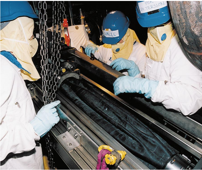
An example of contributing to improved working environments is our cooperation with ABB on the development of a flow stopper. A “rubber bladder” plays an important part in the renovation of a nuclear power plant.
