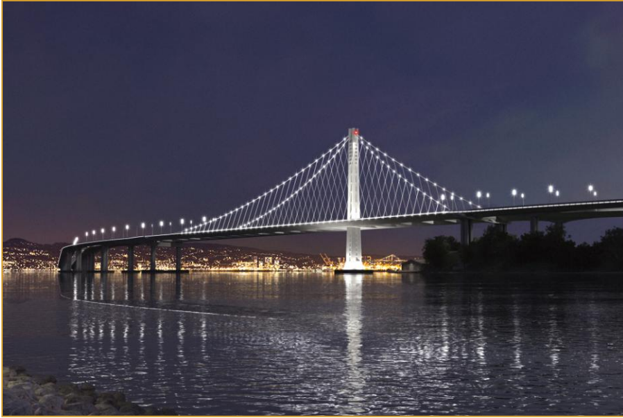
San Francisco Bay Bridge (USA)
