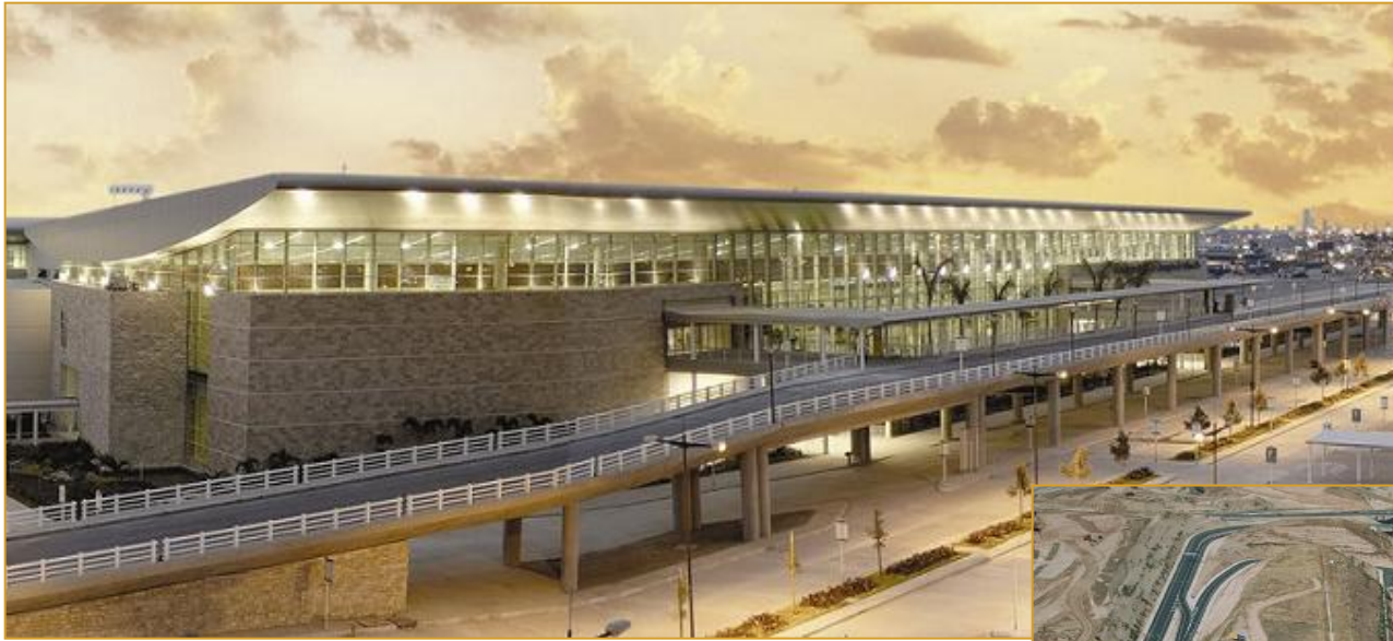
Terminal access to Guayaquil Airport (Ecuador)
