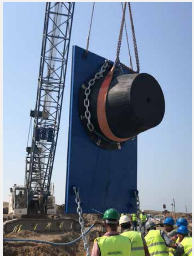
Fender assembly ready for installation on wharf
