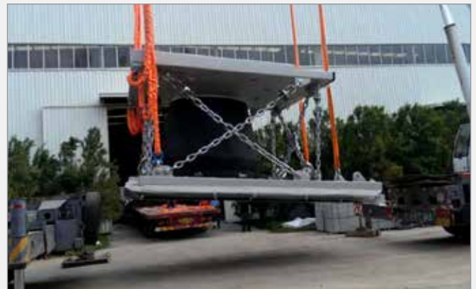
Handling of fender system using rigging equipment with spreader beam
