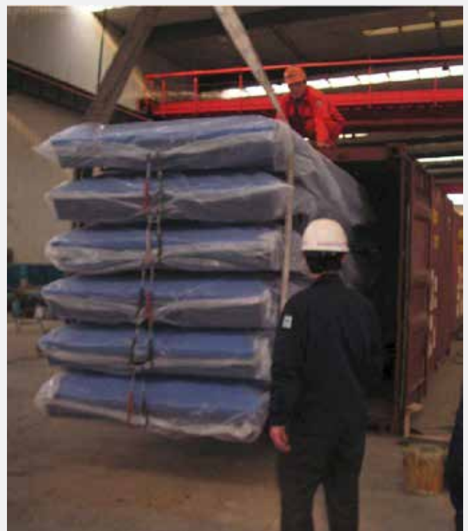
Handling (unloading) frontal frame using crane
