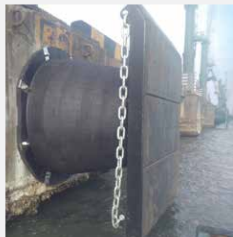
Fastening of fender to wharf
