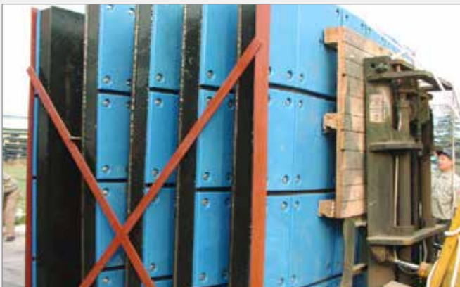
Unloading frontal frame using forklift
