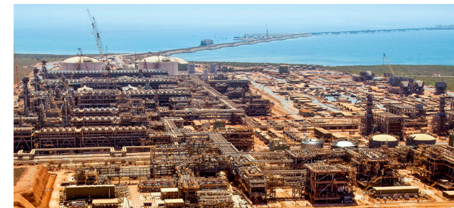
Gorgon LNG installation, Barrow Island, Western Australia
