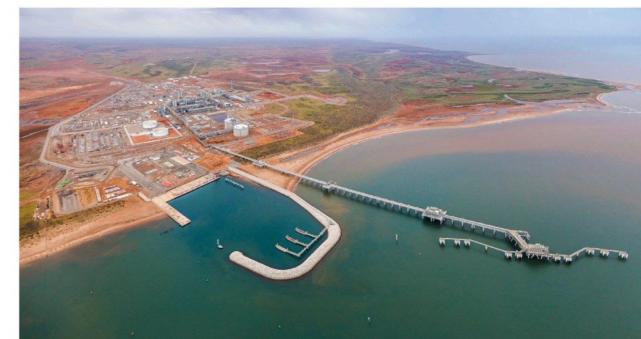
Wheatstone LNG installation, Onslow, Western Australia
