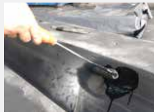
Apply bonding cement
