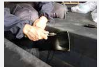
Apply compound layer
