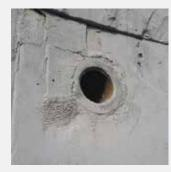
Figure 11 Installed cast-in anchor
