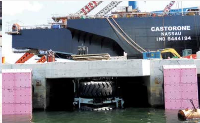
Wheel fenders are widely used on exposed corners to help ships maneuver into berths and narrow channels such as locks and dry-dock entrances.
