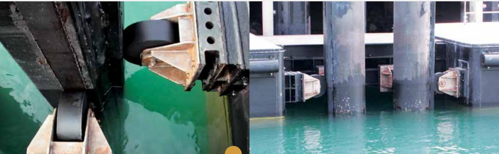
Cushion rollers are used to guide pontoons and floating structures quietly and gently up and down their guide piles.
