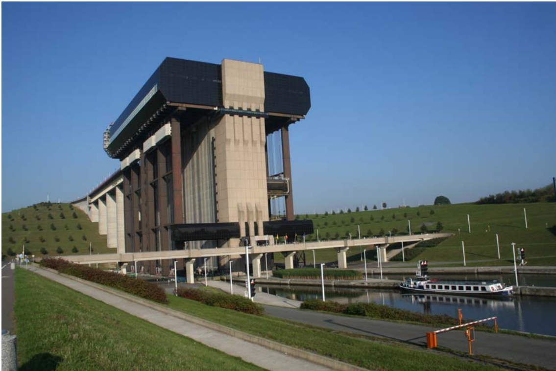
Picture 4: Omega seals between the structures of the canal to the Ship lift of Strépy Thieu - Belgium
