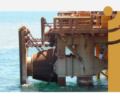
Trelleborg's entire rubber fender range also includes its innovative, patented Slide In, Slide Out fender system, designed to reduce maintenance requirements, by significantly reducing the time and effort taken to complete a fender wear change-out.
