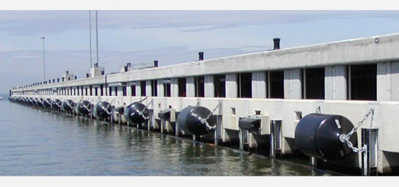
Used in a variety of challenging applications, foam fenders are extremely versatile. Easy to install, they provide a tough, heavy-duty fender solution for in-harbor, off-shore and ship-to-ship applications. Their resilient foam-filled construction provides an unsinkable fender body that permits high energy absorption with relatively low reaction force and hull pressures.
